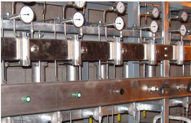
**Total flow rotameters**, which allowed the Lab personnel to quickly view the total sample flow and adjust it to maintain the velocities necessary to keep magnetite and other debris suspended, avoiding sample line pluggage.
