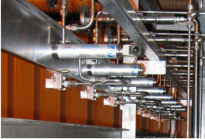
**Problem:** Occasional failure of primary cooling water supply or other factors had occurred in the past, and allowed hot samples to flow into the lab. This had resulted in damage to fragile and expensive instruments.
