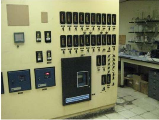
**Problem:** Flow to the analyzers in the lab was variable. The analyzer rotameters required constant adjustment to maintain proper flow.
